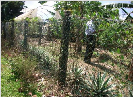
Wire mesh fence establishment
